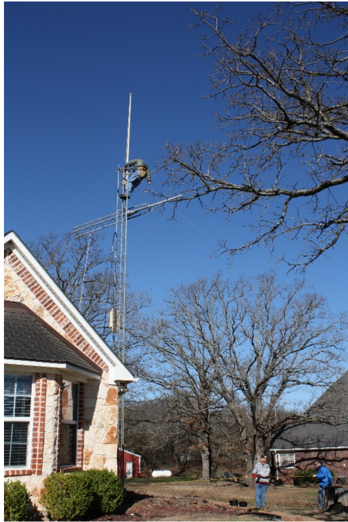
Next we raised and installed the new top section with a rotator and new mast.
