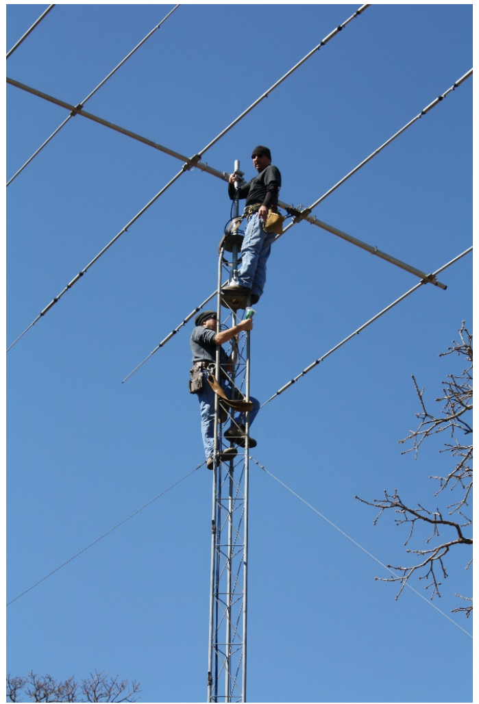
Dan and Ben installing the rotator and coax cables.
